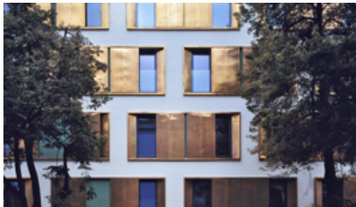
Façade with outside shading elements
